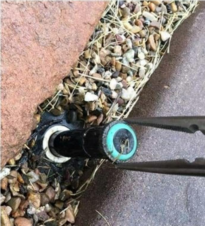
Look how nasty these filters are! Clearly debris is keeping water from flowing through the filter to the nozzle.
